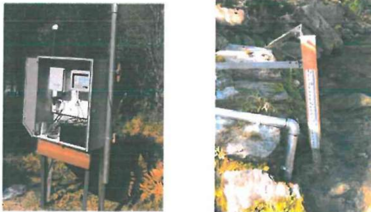
Figure 2. Examples of Design Analysis data logger, bubbler line, and staff gage installation.
